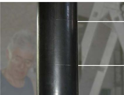
3. The top of each step is marked on the central tube of the staircase.
