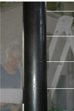
3. The top of each step is marked on the central tube of the staircase.
