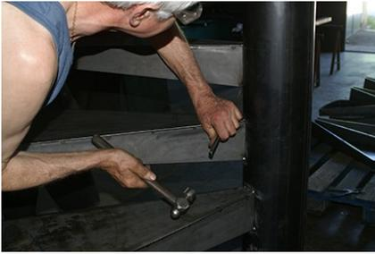
9. With smooth and controlled blows or small pieces of wire the deviation that may be corrected is corrected.
