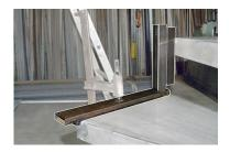
4. A special tool is anchored on the outside of the step. This makes stop at the front and side of the step and tells us where to put the next.
