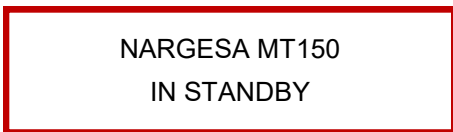
Picture 28. Screen for StandBy on default.
